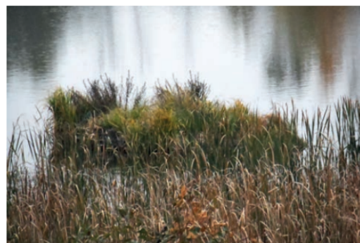
Treatment Wetland is positioned at the outlet of the stormwater pond to remove TSS and avoid clogging the pump. Water has been reused for 3 years to water ball fields in Minnesota.
